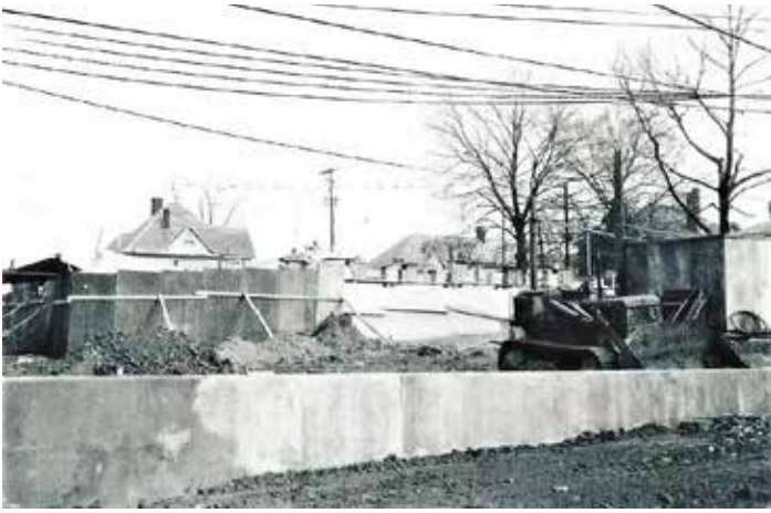
Ohio Power exterior construction taken from parking lot
